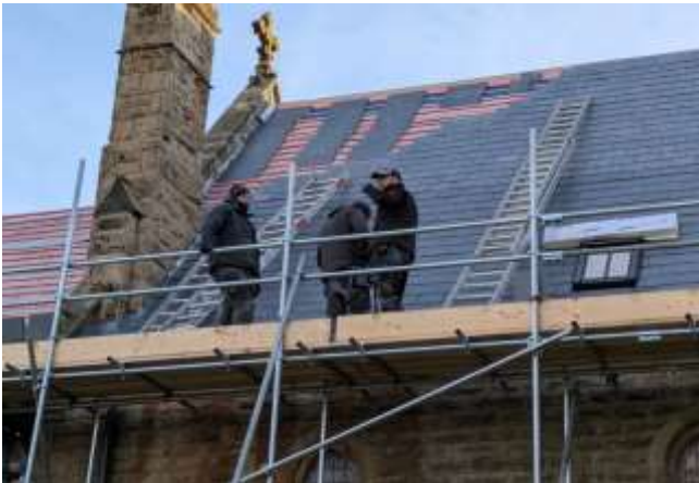
Re-tiling the roof
